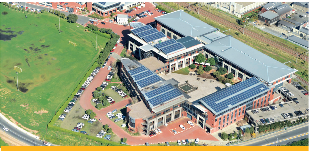
Grid-tied PV system at Black River Park.
